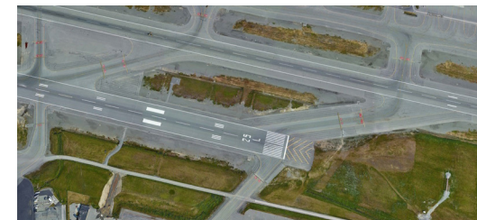
Angled crossfield taxiway geometry does not meet current FAA standards
