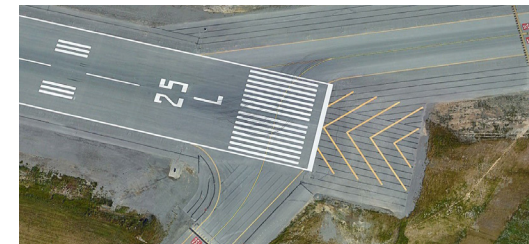
Runway 25L Blast Pad does not meet current FAA standards (length)
